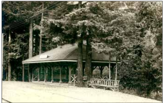
RAILROAD PASSENGER SHELTER AT RIO NIDO. A FAINT INSCRIPTION ON THE IMAGE READS, "BELDEN & UPP PHOTO," BUT BACK IMPRINT (ABOVE) ON THE CARD REVEALS NEGATIVE WAS REPRINTED BY LARK & WARNE.
