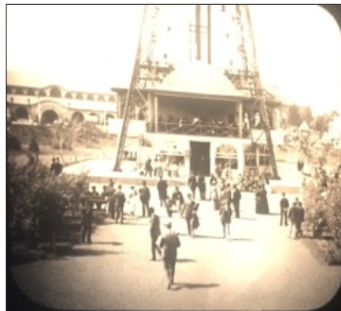
BASE OF THE ELECTRIC TOWER
