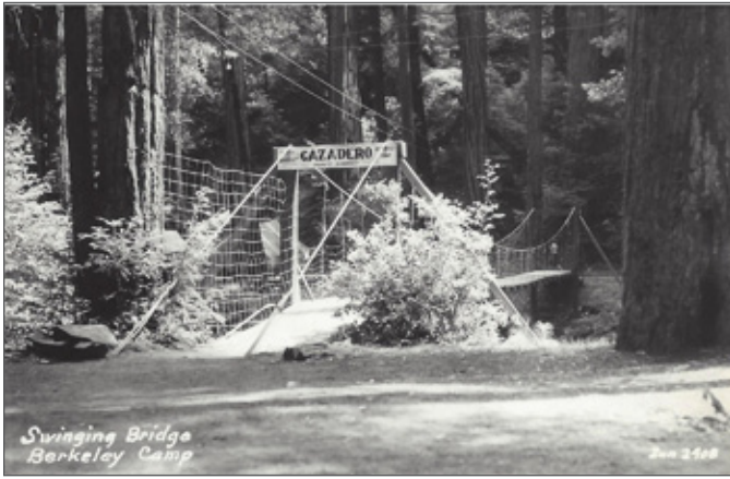
THE CITY OF BERKELEY PURCHASED PROPERTY IN CAZADERO IN 1929 FOR USE AS A SUMMER CAMP, AND INSTALLED THIS SUSPENSION BRIDGE OVER AUSTIN CREEK. IT WAS CALLED SWINGING BECAUSE KIDS JUMPED UP AND DOWN TO GET IT MOVING. IT CURRENTLY PROVIDES ACCESS TO CAZADERO PERFORMING ARTS MUSIC CAMP. [ZAN 2408, 1946; PRODUCTION TOTAL 1200]
