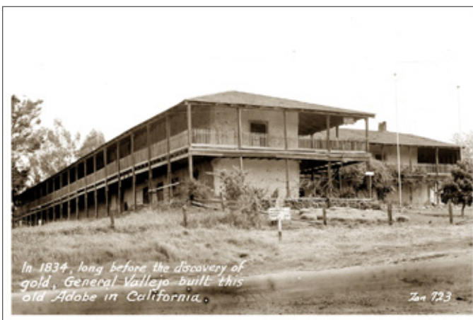
GENERAL M.G. VALLEJO BUILT THIS HUGE 2-STORY STRUCTURE TO SERVE AS HEADQUARTERS FOR HIS 66,000-ACRE LIVESTOCK RANCH DURING 1836-46. CONSTRUCTED OF ADOBE BRICK AND REDWOOD, AND TYPICAL OF HISPANIC ARCHITECTURE, IT SITS 6 MILES EAST OF PENNGROVE. [ZAN 723, 1941]
