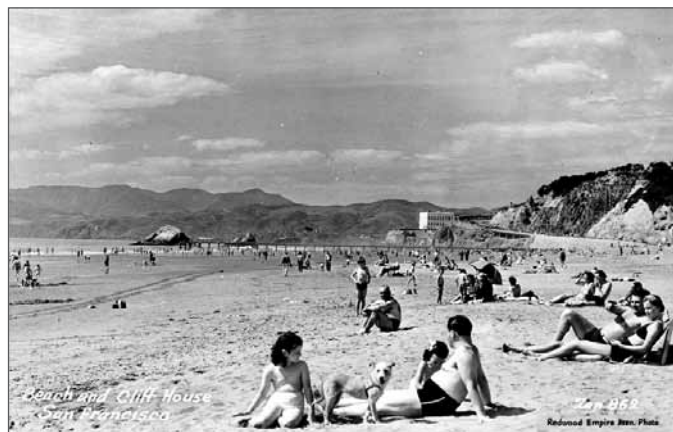
EXCEPT FOR REMOVAL OF THE LURLINE PIER, THE VIEW LOOKING NORTH TOWARD THE CLIFF HOUSE REMAINS BASICALLY UNCHANGED AFTER 70 YEARS. [ZAN 862, REA PHOTO]
