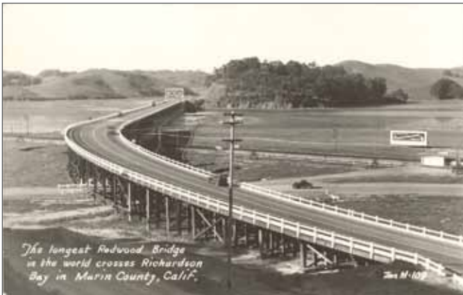
ROUTING HIGHWAY 101 THROUGH MARIN COUNTY CULMINATED WITH NOVEMBER 1931 COMPLETION OF THIS REDWOOD BRIDGE, A QUARTER-MILE SPAN OVER RICHARDSON BAY. BUILT TO LAST A CENTURY, IT WAS REPLACED WITH CONCRETE AND STEEL IN 1956. [ZAN M-109, C. 1933]
