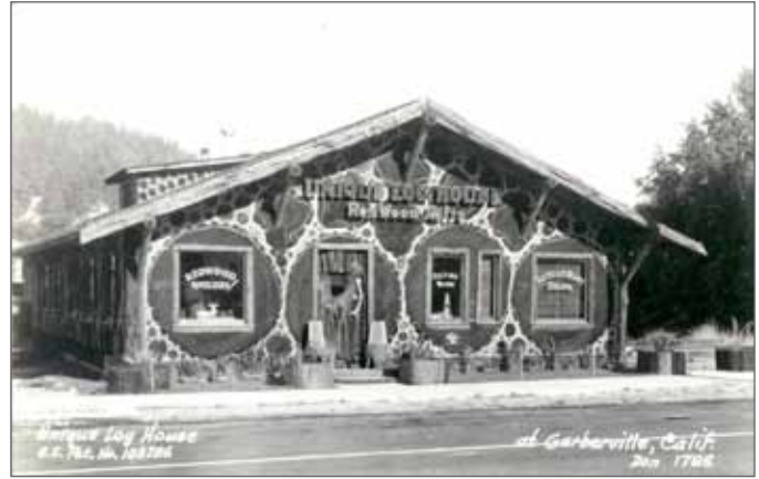
THE UNIQUE LOG HOUSE GIFT SHOP AT GARBERVILLE WAS UNIQUE BECAUSE ITS WALLS WERE CONSTRUCTED ENTIRELY OF CROSS-CUT REDWOOD LOG SECTIONS. NOTE DESIGN PATENT NUMBER AT LOWER LEFT. [ZAN 1786, 1937]
