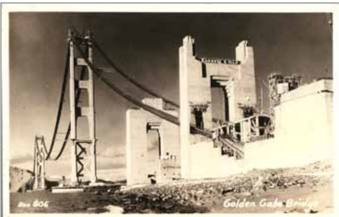
IN NOVEMBER 1932, BARRETT & HILP OF SAN FRANCISCO WERE AWARDED $2 MILLION IN CONTRACTS TO BUILD CONCRETE ANCHORAGES AND TO PAVE THE ROADWAY FOR THE GOLDEN GATE BRIDGE. [ZAN 806, C. 1936]
