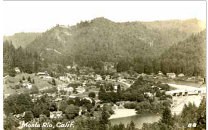
THIS VIEW CARD WAS LIKELY PRODUCED FOR MONTE RIO MERCHANT SIDNEY A. BARTLETT. THE CONCRETE HIGHWAY BRIDGE AT RIGHT, DEDICATED IN MARCH 1935, IS CURRENTLY SCHEDULED FOR REPLACEMENT. [88, PHOTO POSTCARD MADE BY ZAN]
