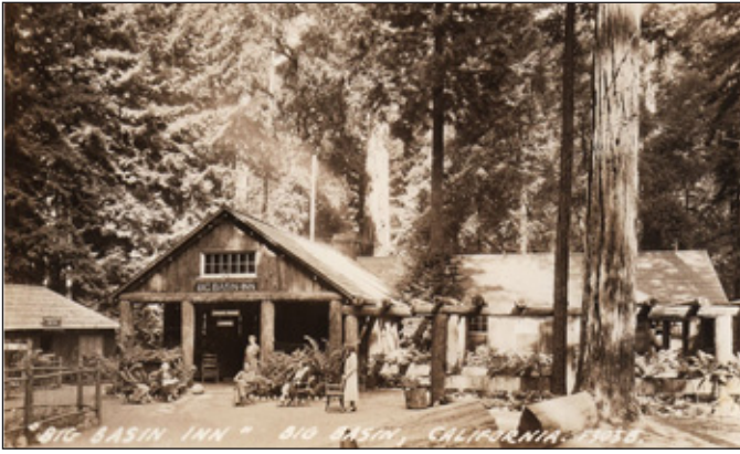
BIG BASIN INN WAS A MANAGEMENT AND PUBLIC USE BUILDING FOR 50 RENTAL CABINS IN THE GOVERNOR'S CAMP AREA. CONSTRUCTION STARTED IN 1911 AND WAS KNOWN AS REDWOOD PARK INN UNTIL 1928. FULMER PHOTO, C. 1932 (F303B PHOTO POSTCARD)
