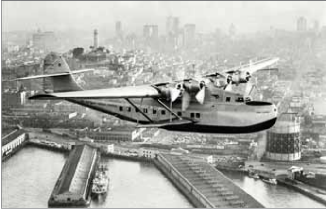
PAN AMERICAN CHINA CLIPPER, ABOVE THE EXPANDING GAS STORAGE TANK
