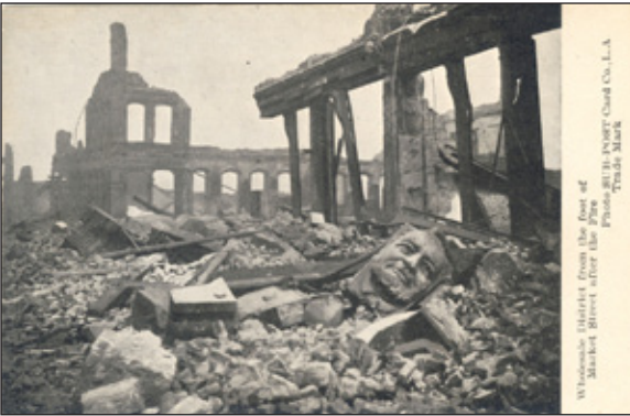
EARTHQUAKE AND FIRE DAMAGE AT MARKET AND FREMONT STREETS. WINE MERCHANT SAM LACHMAN'S STONE FACE SITS IN THE RUBBLE, BRAVELY FACING DISASTER.
