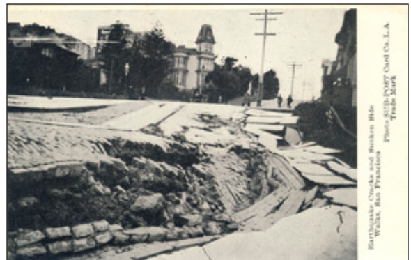
SUNKEN STREET AND SIDEWALK IN SAN FRANCISCO DISTRICT THAT ESCAPED FIRE.
