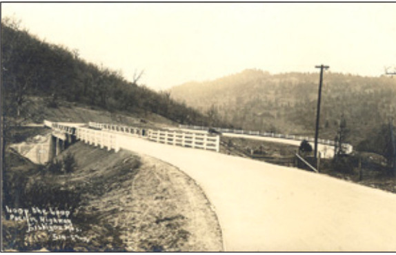
STEINMAN BRIDGE AND 360° UNDERPASS DUBBED "LOOP THE LOOP" BY PHOTOGRAPHER FRANK PATTERSON, c. 1925.
