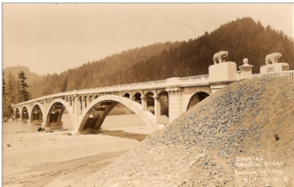
854—DOUGLAS BRIDGE, REDWOOD HWY, WASHED AWAY 1964.
