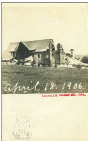
TUMBLING STONE RUINS OF THE CATHOLIC CHURCH. RESTORED STEEPLE AT RIGHT INDICATES PHOTO TAKEN WEEKS AFTER THE INSCRIBED DATE.
