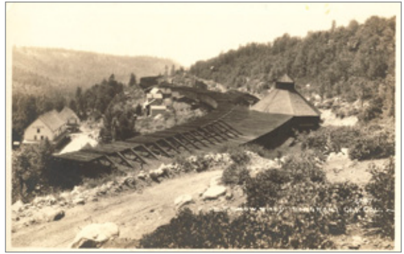
ALLEN HOTEL AND SOUTHERN PACIFIC RAILROAD'S SNOW SHED AT EMIGRANT GAP, A SMALL COMMUNITY ON THE OTHER SIDE OF THE RIDGE FROM LOOKOUT POINT.
