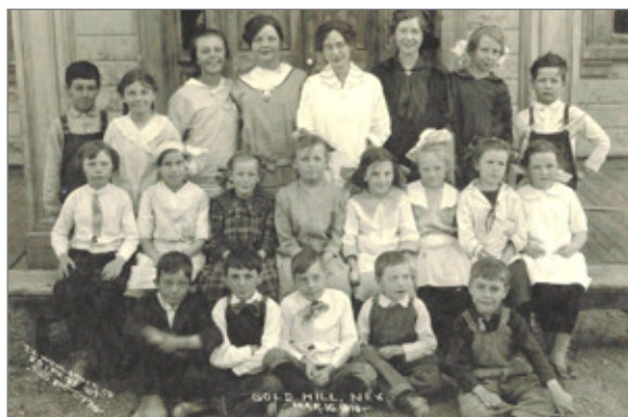
GOLD HILL, NEVADA SCHOOL T. C. WOHLBRUCK CO., SAN FRANCISCO, MARCH 16, 1916.
