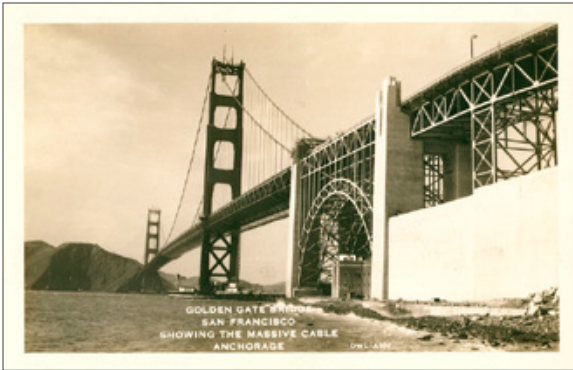
A102 SOUTHERN ANCHORAGE OF GOLDEN GATE BRIDGE ARCHING OVER FORT POINT
