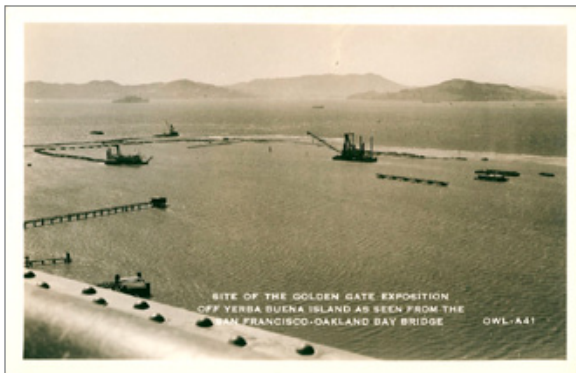
A41 DREDGES AND BARGES DURING FIRST STAGES OF CREATING TREASURE ISLAND.
