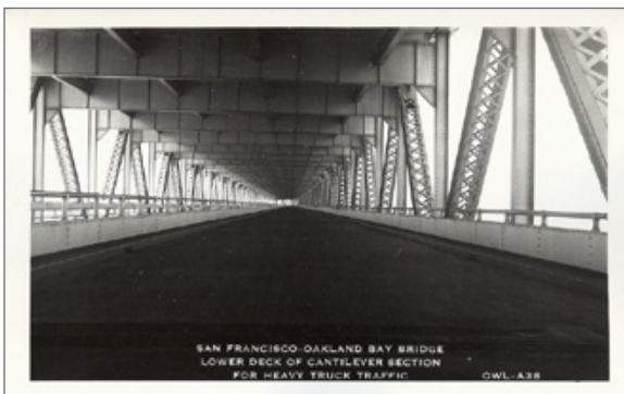
A38 LOWER DECK OF CANTILEVER SECTION OF BAY BRIDGE, ALMOST READY FOR TRUCK TRAVEL.
