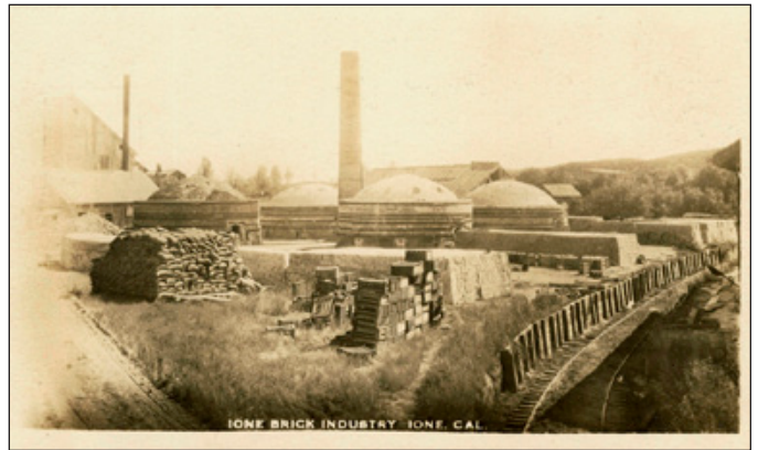
This factory in Ione must have reminded John Bowers of laboring in his brother's brickyard in Topeka as a teenager.
