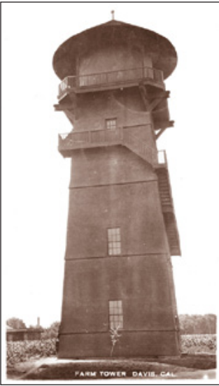
University of California at Davis. The 60-foot redwood-shingled water tower was built in 1908, south of where the Shields Library now stands. Post-marked October 1911.
