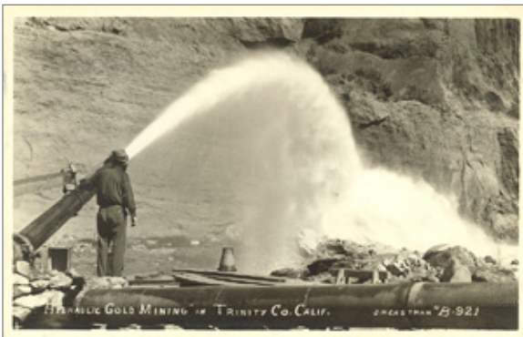
J. H. EASTMAN — HYDRAULIC GOLD MINING IN TRINITY COUNTY, 1939
