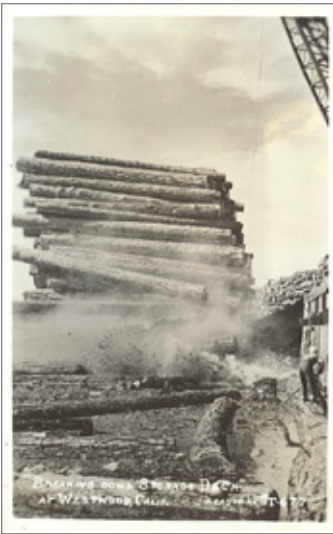
J. H. EASTMAN — BREAKING DOWN STORAGE DECK AT WESTWOOD, 1943
