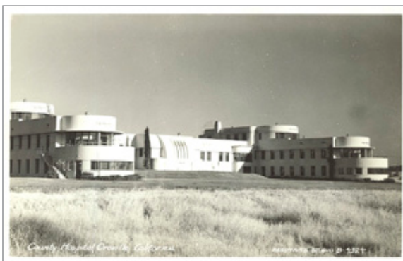
EASTMAN'S STUDIO — BUTTE COUNTY HOSPITAL, OROVILLE, 1946
