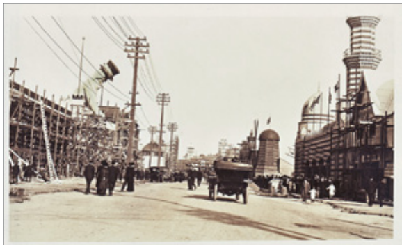
THE ZONE UNDER CONSTRUCTION
