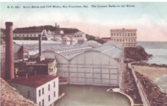
EARLY VIEW FROM NORTH WITH 1909 CLIFF HOUSE ADDED
