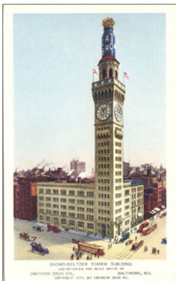
Bromo-Seltzer Tower Bldg., Baltimore 1911
