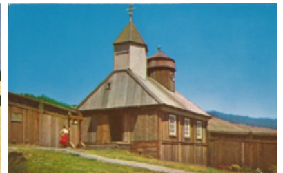
AFTER 1970 - THREE WINDOWS
