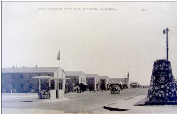
CAMP STONEMAN, PITTSBURG CA — POW TRANSFER POINT
