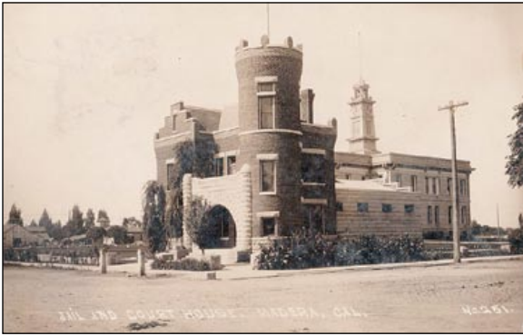
MADERA COUNTY JAIL — BESAW
