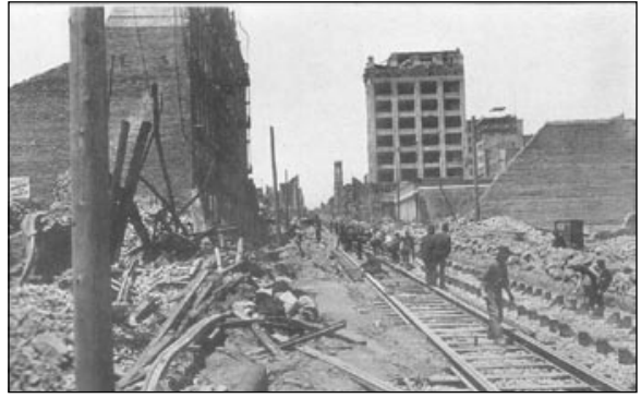
REMOVING CABLES AND INSTALLING TROLLEY TRACKS ON SUTTER
