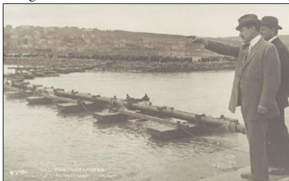
SUCTION DREDGING AT HARBOR VIEW
