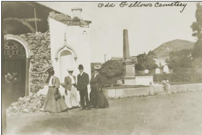
1906 QUAKE DAMAGE BY COLUMBARIUM, CALIFORNIA HISTORICAL SOCIETY
