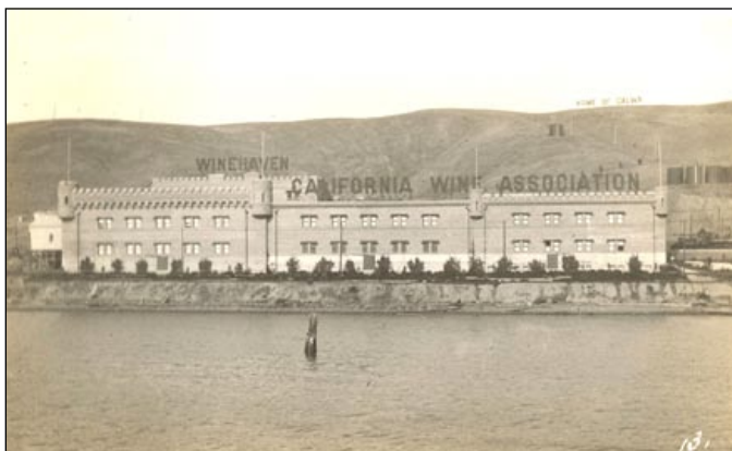
Decorative parapet and turrets are clearly visible on the storage depot in this circa 1910 real photo. A sign reading, "Home of Calwa" has been placed on the crest of the hill, and some trees and shrubs planted.
