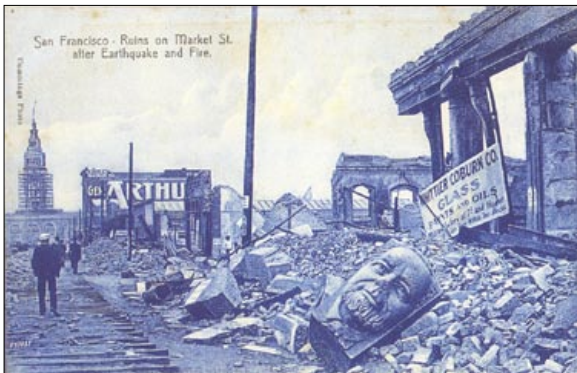
View of San Francisco ruins featuring Samuel Lachman's stone face that fell 60 feet on April 18, 1906. Oliver G. Cummings photo looking east on Market toward Ferry Building taken May-June 1906. Pacific Novelty Co. postcard published circa mid-1907. (Glenn Koch collection)
