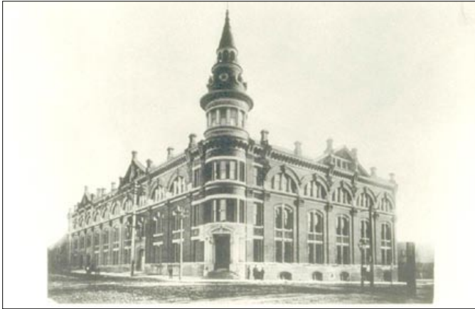
Kohler & Frohling wine depot, Second and Folsom, at completion in early 1890. The “castle” served as California Wine Association headquarters 1894–1899. (Courtesy Bancroft Library).
