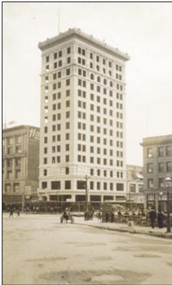
David Hewes Building, 995-997 Market, under construction 1908, savagely remodeled with an aluminium and glass skin in the 1960s.
