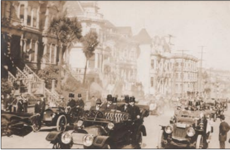
TAFT MOTORCADE, 900 BLOCK OF STEINER STREET, BETWEEN MC ALLISTER AND FULTON, LOOKING MUCH THE SAME TODAY.
